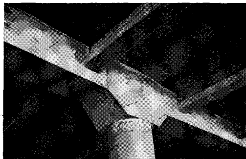
Fig. 14—Close-up photograph of the completed composite connection between joists, beams, and a corbel.
