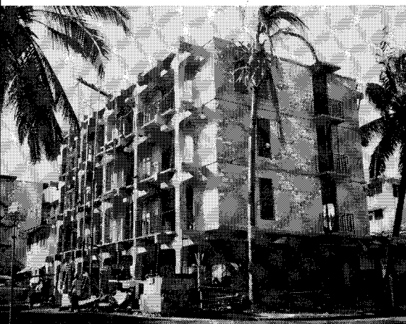
Fig. 22—Nearly completed building five weeks after lifting first column tree.
