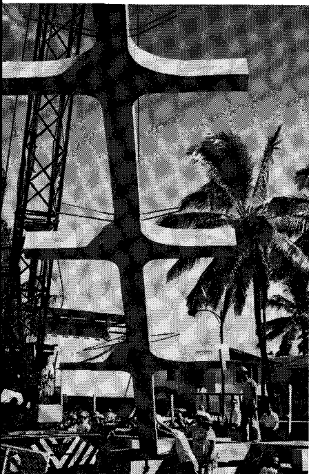
Fig. 20—Erecting first precast column tree.
